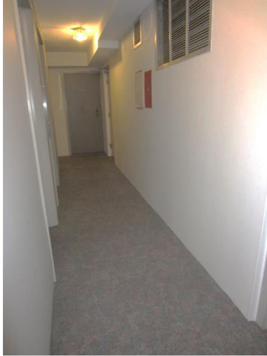
Image 30. Typical Hallway Finishes
