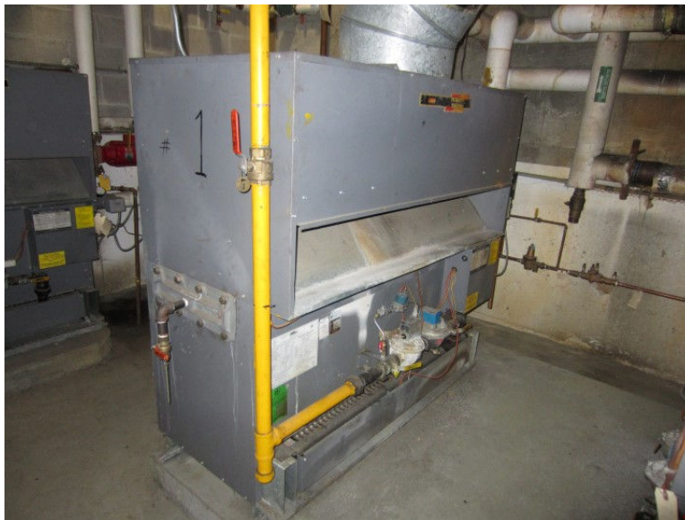
Image 45. Natural Gas Boiler
