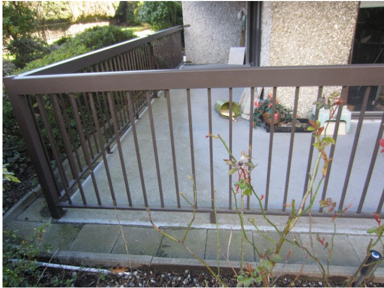
Image 11. Typical Painted Concrete
