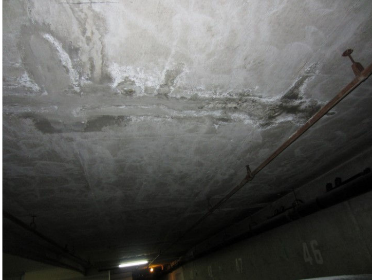
Image 1. Repair Crack Actively Leaking
