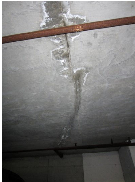
Image 2. Crack in Ceiling
