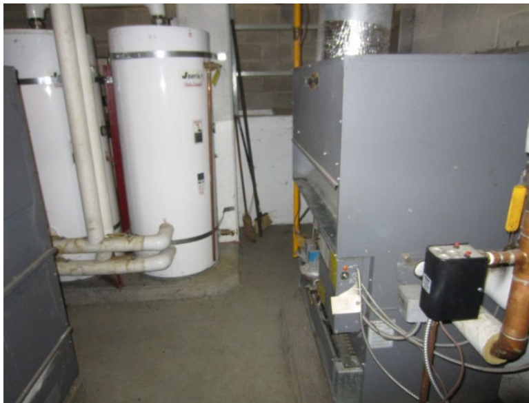
Image 39. Boiler and Hot Water Tanks
