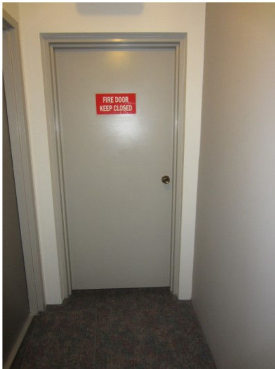
Image 20. Exit, Fire Rated Doors
