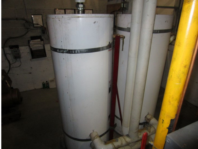
Image 38. Hot Water Tanks
