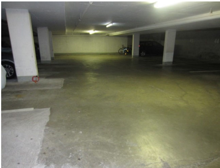
Image 47. Underground Garage Fixtures
