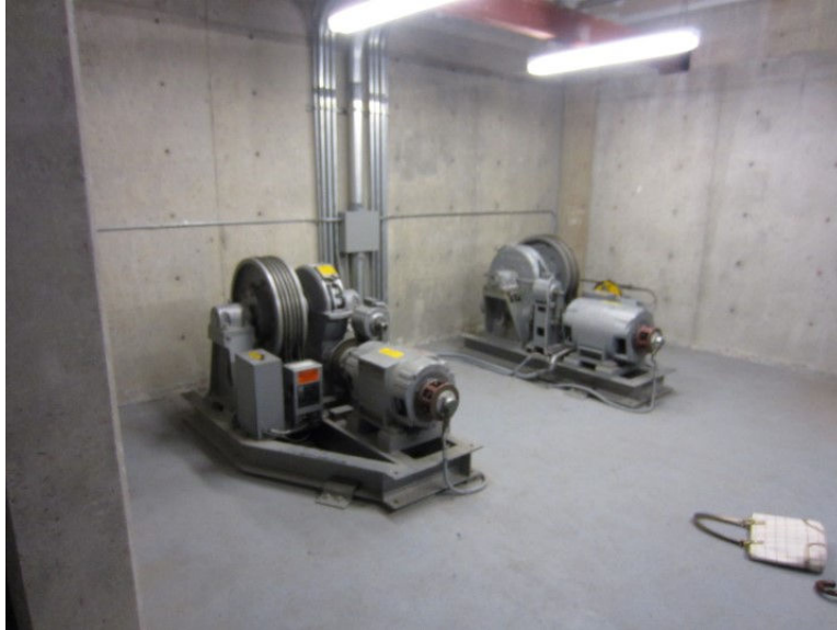
Image 36. Traction Elevator Sheaves
