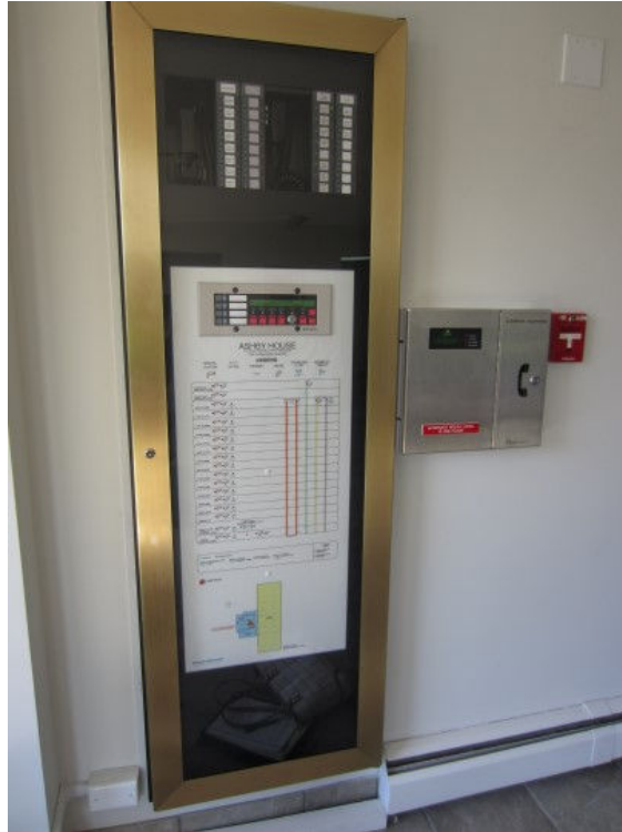
Image 42. Fire Alarm Display Panel
