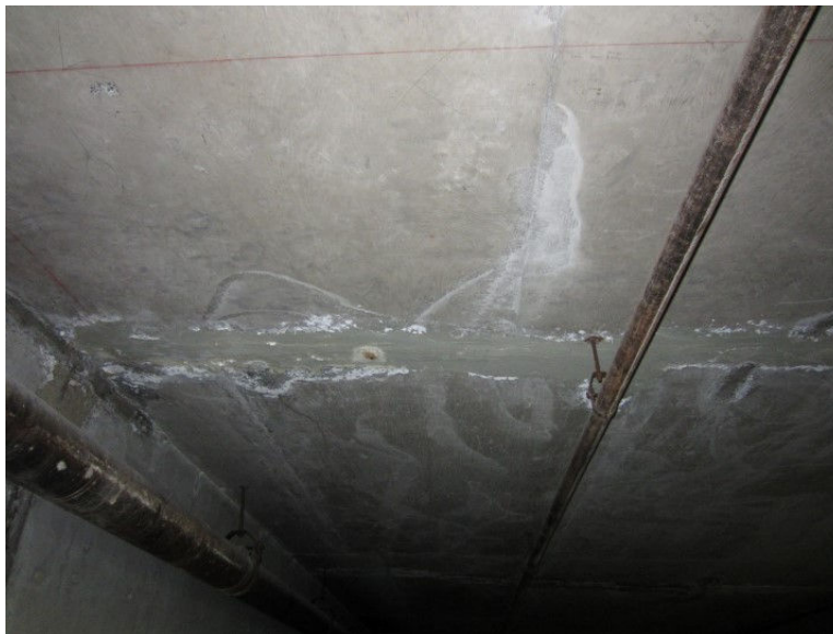
Image 4. Repaired Crack in Ceiling
