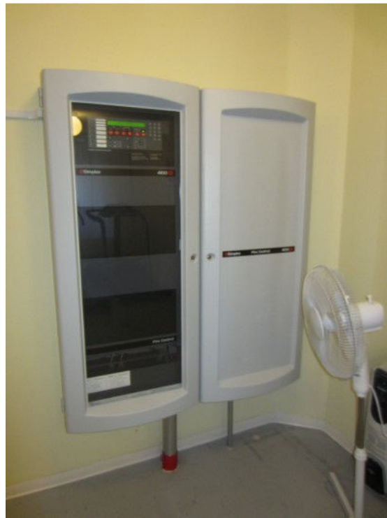
Image 43. Fire Alarm Panel
