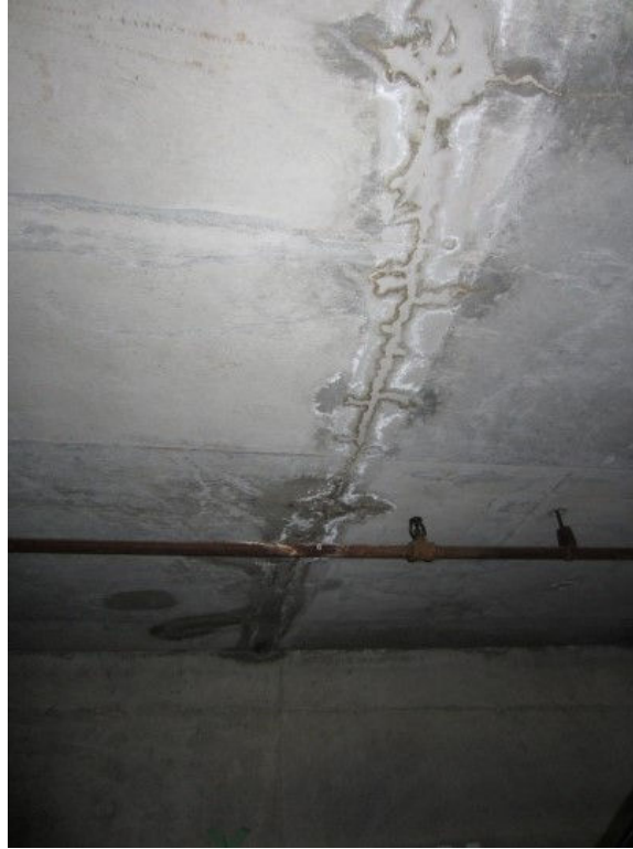
Image 3. Crack in Ceiling
